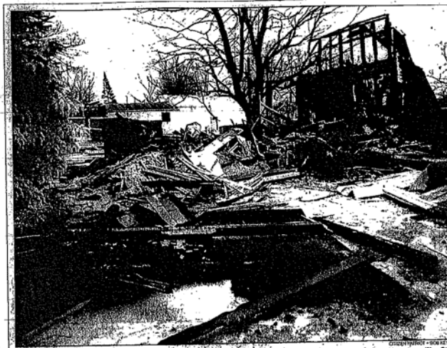
The home at 113 Austin Road remains a pile of rubble today. The white building in the background is the Napoleon Fire Station. A wreath to victims Ralph and Bernice Davis can be seen at right.
